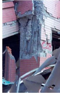
Figure 30: Lack of Confinement at Column Head
