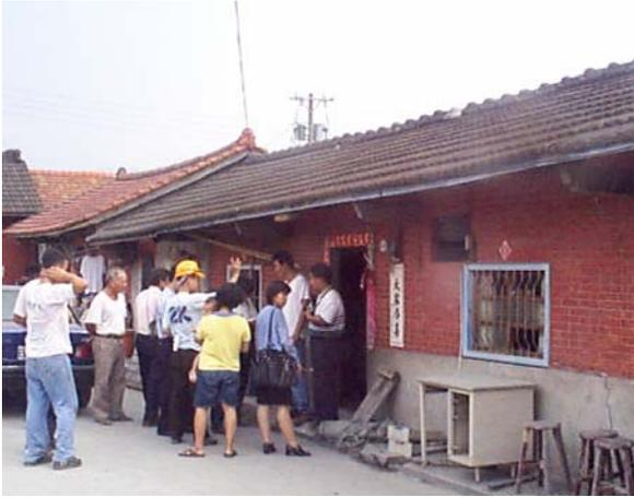
Figure 8: Single floor tiled roof house suffers settlement following liquefaction of sub-strata
