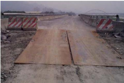
Figure 45: Settlement of the approach roads relative to the bridge deck
