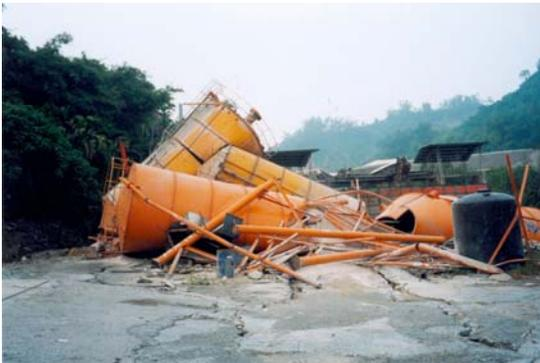
Figure 33: Collapsed Silos
