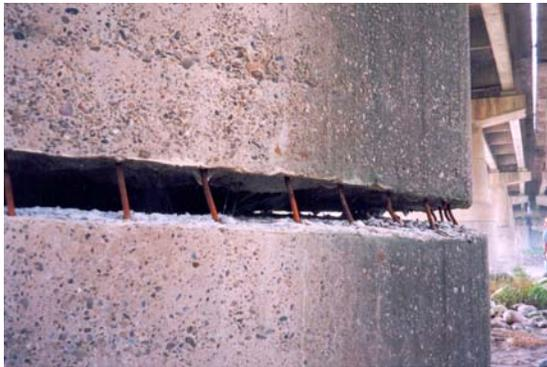
Figure 38: Close Up of Bridge Pier Reinforcement
