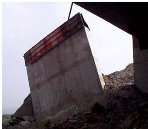
Figure 42: Bridge abutment completely destroyed
