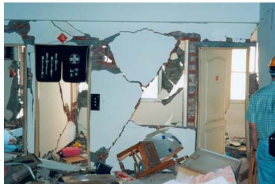
Figure 28: Shear Cracking of Internal Walls
