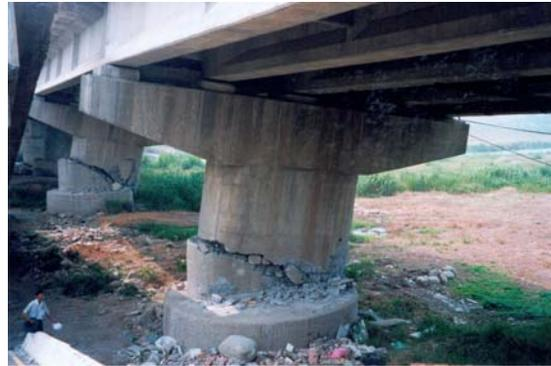
Figure 37: Shear and Transverse Displacement of Bridge Piers
