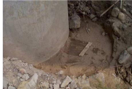
Figure 44: Close up view at the base of the pier showing the original mark of the pier before lateral spreading
