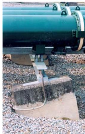
Figure 35: Pipeline Settlement Through Ground Liquefaction
