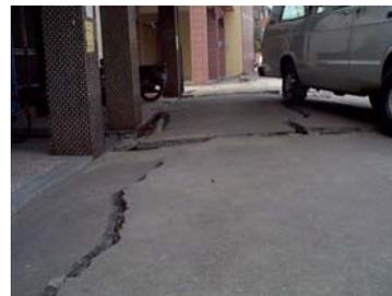
Figure 15: Settlement of the ground floor relative to road level
