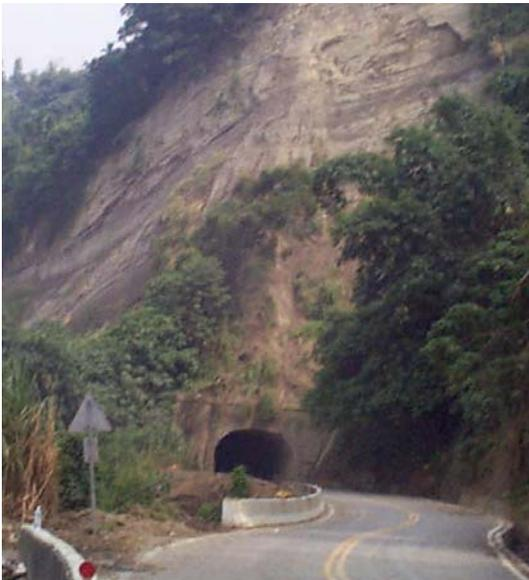
Figure 21: Tunnel located in the side of a hill with landslides at the surface
