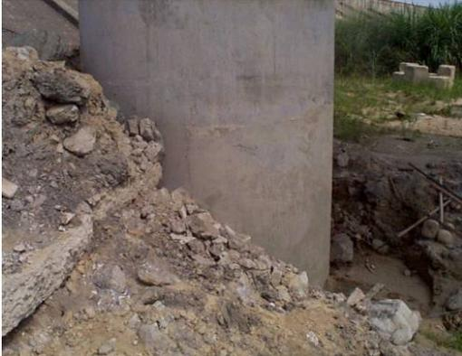
Figure 43: Soil flow obstructed by the pier causes a ground heave behind the pier
