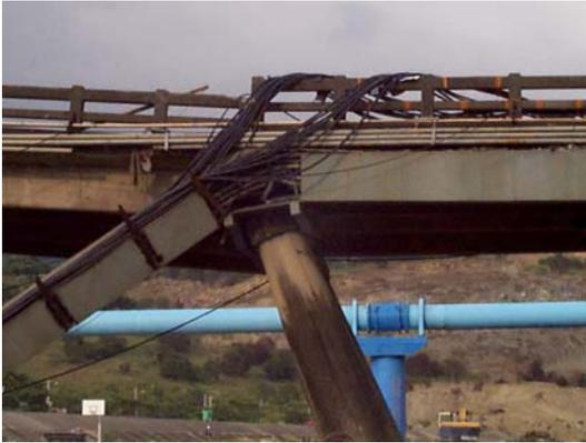
Figure 39: Rotation of the old bridge piers due to deck movements
