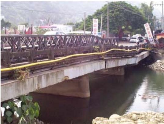
Figure 5: Where fault movements were smaller, bridges survived collapse
