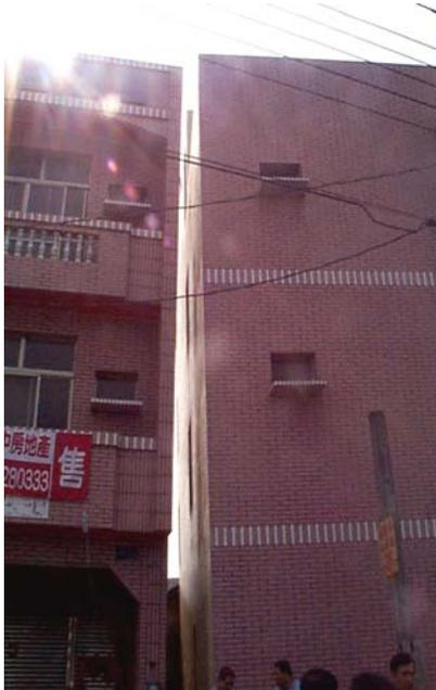
Figure 14: Building rotation due to differential settlement following liquefaction of the foundation soil
