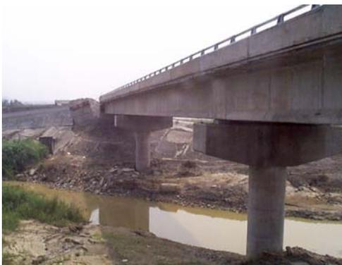
Figure 41: Overview of the bridge and the piers, the abutment on the far side was destroyed as seen in Figure 42
