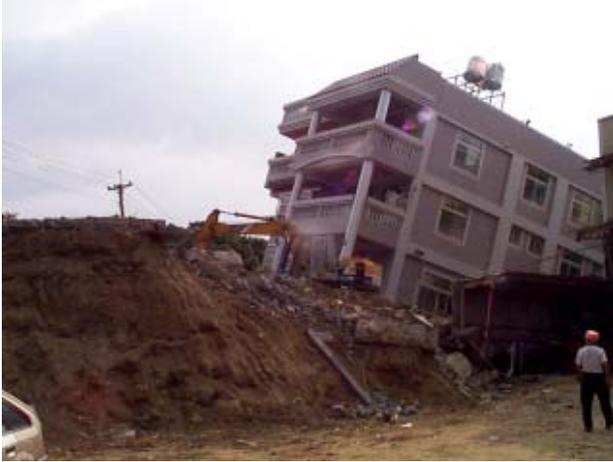
Figure 1: Fault movement caused this spectacular lift of this building that straddled across the fault
