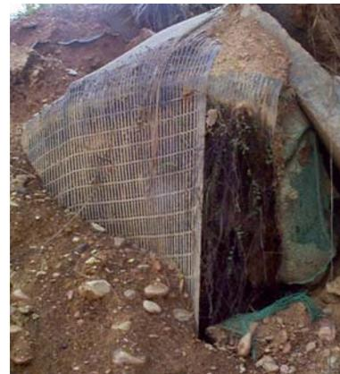
Figure 25: The wrapping of the Geotextile around Geonet gabions filled with was pulled out en bloc
