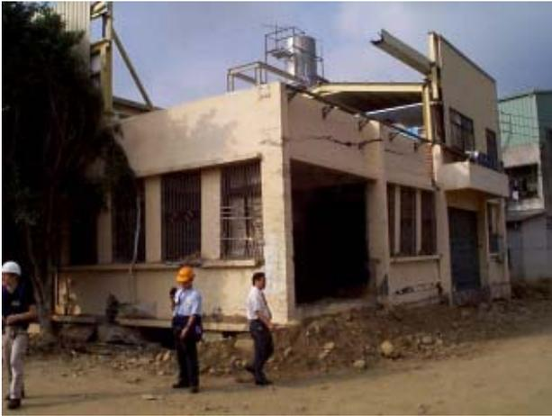
Figure 2: The building next to the one seen in the figure before suffered damage but survived without collapse
