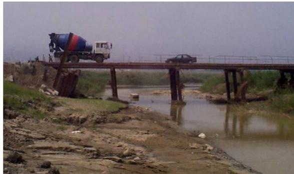
Figure 46: Precarious rotations of the old bridge piers, pressed into action to ferry materials to repair the new bridge abutment
