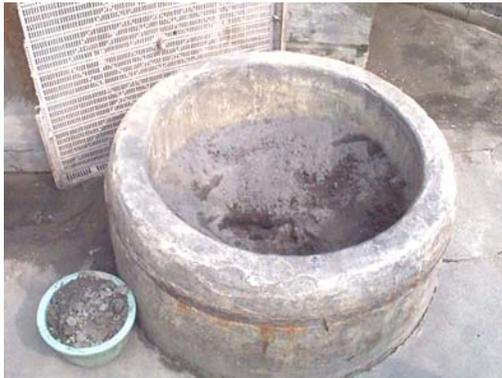
Figure 10: Well filled by liquefied soil
