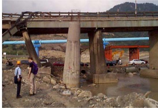
Figure 40: The new piers with no bridge deck suffered rotation in the opposite direction
