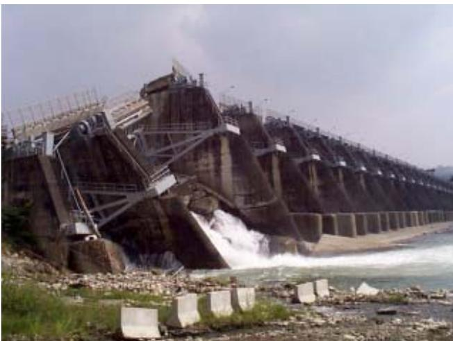
Figure 6: Failure of the dam due to fault movement (right hand side was uplifted by the earthquake)
