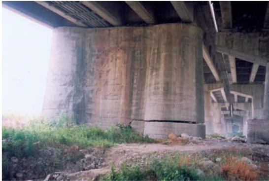
Figure 36: Bridge Pier Failure from Transverse Acceleration
