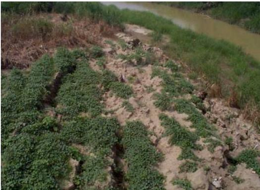
Figure 17: Lateral spreading of the slopes parallel to abutments showing deep tensile cracks
