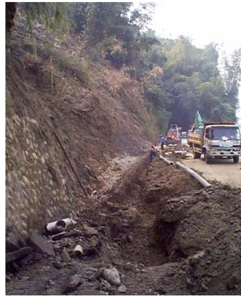
Figure 22: Landslides caused failure of the lifelines laid next to the roadway
