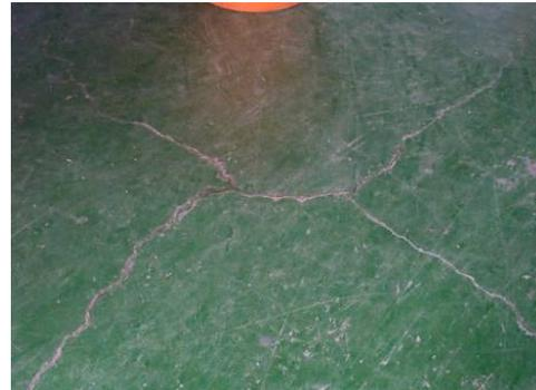
Figure 13: Yield lines in floor slab
