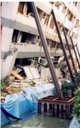
Figure 31: Soft Storey Failure
