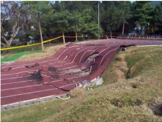
Figure 3: The athletic track at Wu Fang School suffered badly due to fault movements
