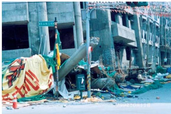
Figure 32: Soft Storey Failure
