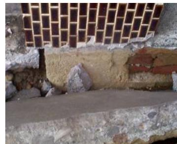
Figure 16: Settlement of a column at the foundation
