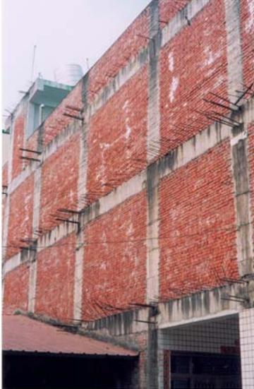
Figure 26: Typical urban construction of a reinforced concrete frame with brick infill
