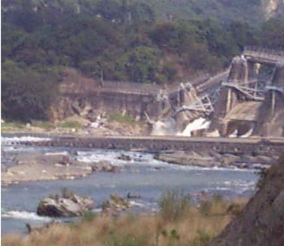
Figure 7: Left hand edge of the dam which indicates the original level of the dam crest
