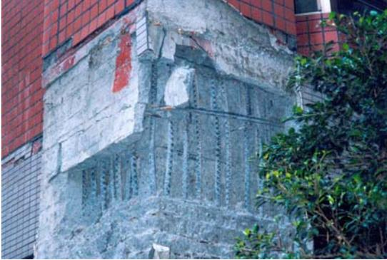
Figure 29: Loss of Cover at Beam/Column Interface
