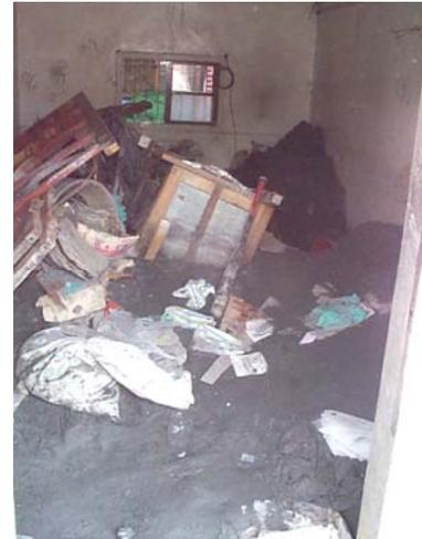
Figure 9: A view inside the house showing the inflow of sub-strata filling the room and lifting the furniture
