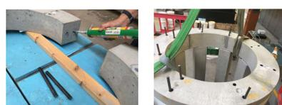
All elements were connected with steel dowels and epoxy resin grout
