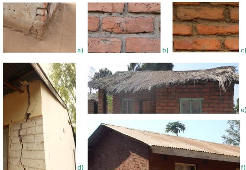
*Figure 4: a) poor connection at the bottom of walls; b) local masonry made of fired brick with cement mortar; c) local masonry made of fired brick with mud mortar; d) complete disconnections between adjacent walls due to poor connection e) thatched roof; and f) metallic sheet roof. (Adapted from Novelli et al 2019-c).*
