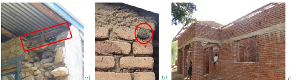
Figure 14: a) Timber wall plate of rectangular section, b) timber wall plate of circular section, and c) concrete ring beam. (Novelli et al. 2019-a).
