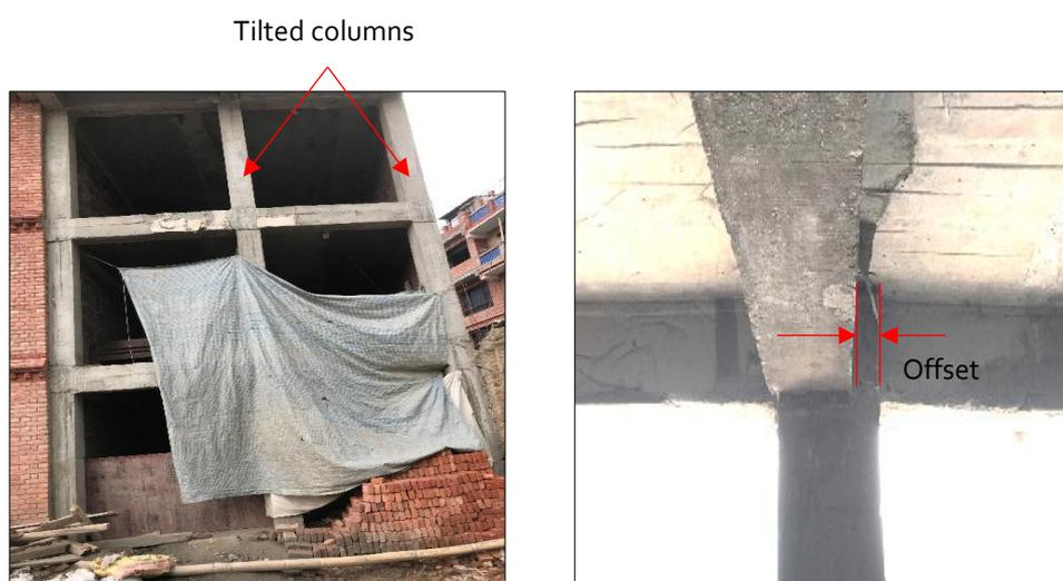
Figure 15. An under-construction RC framed building with tilted columns (left) and poor workmanship of a joint resulting in offset of beams (right) (Photos from Bhaktapur district).
