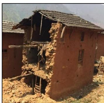
(b) Complete out-of-plane collapse (Photo: Build Change)
