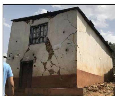
Figure 6. Main failure mechanisms of PRE-SMM typology observed in the 2015 Nepal earthquake.
