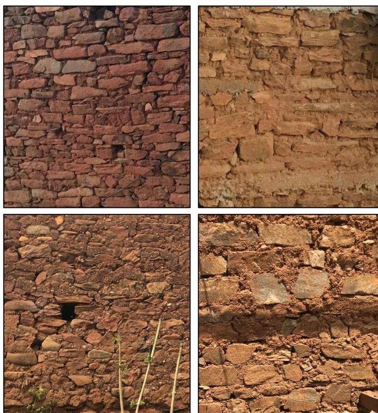
Figure 22. Stone masonry bond pattern from 4 different Nepalese SMM buildings.
