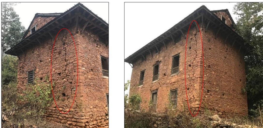
Figure 43. Actual damage due to the 2015 earthquake in the case study PRE-SMM building from Sindhupalchowk district. Vertical separation cracks have a maximum width of about 20 mm.
