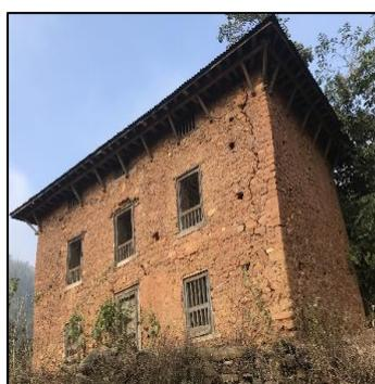
(a) Separation of short wall at cross-wall connection
