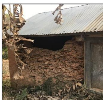
(e) Out-of-plane bulging and debonding
