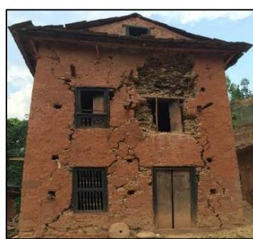
(d) Shear damage in in-plane walls with openings
