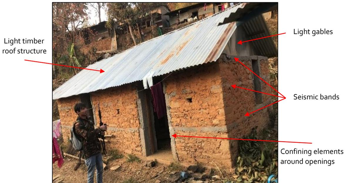
Figure 26. Construction characteristics of typical POST-SMM buildings (Photo from Sindhupalchowk district).
